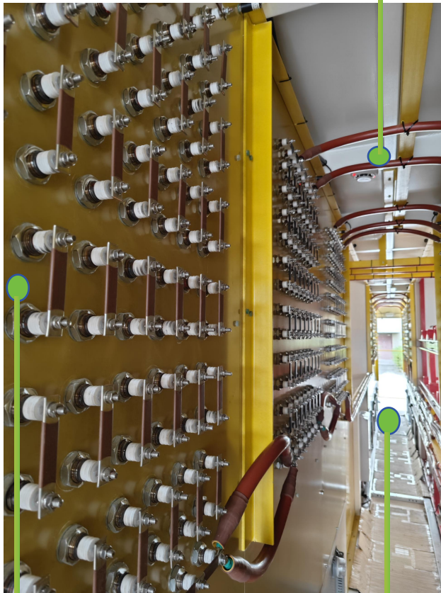
Resistor holding board Material:Epoxy resin
