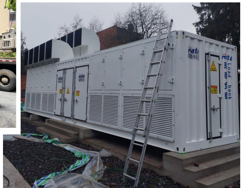
Installation at customer's site
